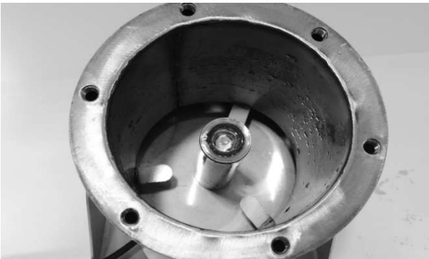
Rinse and scrub clean any dirt inside the chamber
