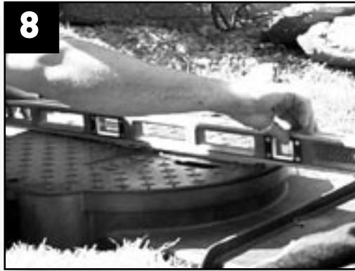
Level the unit front to back and side to side. Make the front edge  $\frac{1}{4}$ " lower than the back edge. **Check water level once again.**
