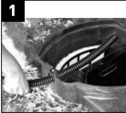
1 Slide hose through pre-cut hole in Skimmerfilter.™
