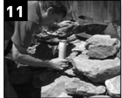
**11** Black foam fills voids in the rockwork and forces water to run over the rocks instead of beneath and between them.
