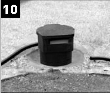
**10** Drain filter before proceeding. Place filter in previously determined site prior to excavation. Bury in position to a depth of 12". As the digging proceeds the excavated soil will be piled around the filter to create the waterfall and stream foundations.
