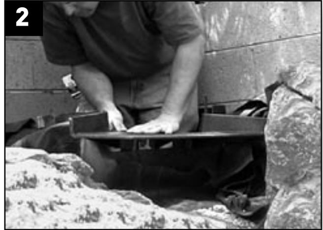
**2** Slide waterfall weir into place. Ensure that the weir seal is firmly compressed between the weir and filter chamber, with flat side of seal facing toward the filter body.
