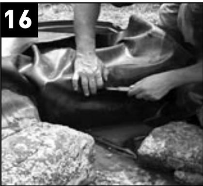
**16** **A)** Make a 3" wide incision through the centered liner ¾" below the top of the Skimmerfilter™ opening.
