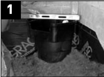
**1** Level the soil in the area where the filter is to be placed. Use blocks to add height to the waterfall. Place filter and level the unit front to back and side to side.
