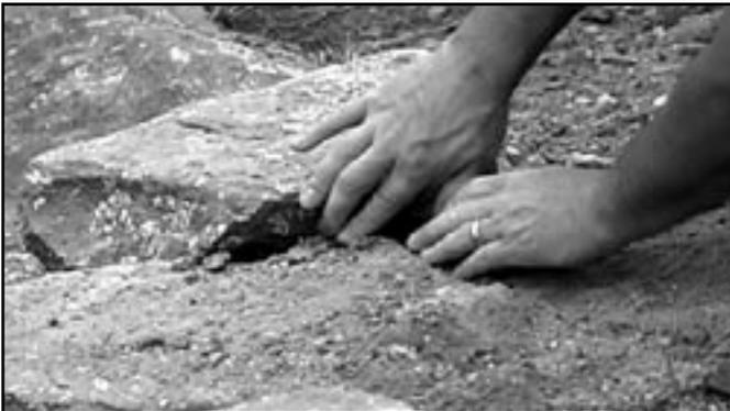
With the pond filled the weight of water will cause the liner to settle. Liner can be trimmed and hidden in the backfill at this time. Do not allow soil to contact water.
