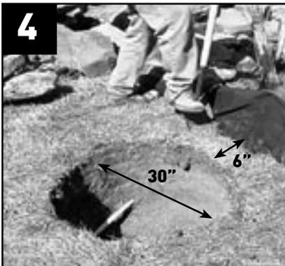
6" back from the coping shelf, dig a round hole measuring 30" across, with a depth of 17" below the marked water line. Dig the front of the hole ¼" deeper than the back to compensate for settling.
