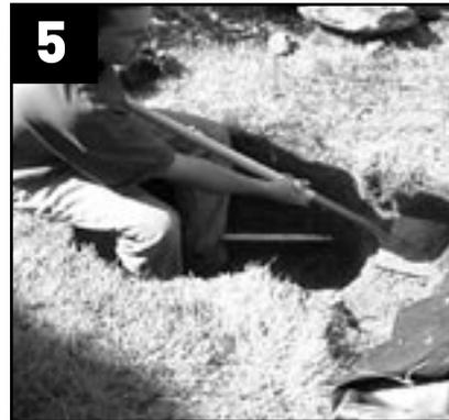
Dig a channel 7" below the water line, measuring 24" wide, from the hole to the pond. The Skimmerfilter.™ neck rests on this channel. Compact and level the bottom of excavation. Do not dig too deeply or the soil may settle unevenly.
