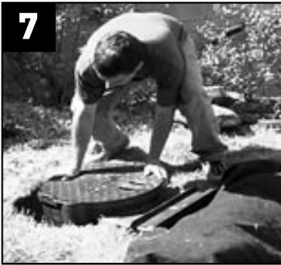
Verify that the face of the Skimmerfilter™ is flush with the back wall of the lined coping shelf. Adjust placement, if necessary.
