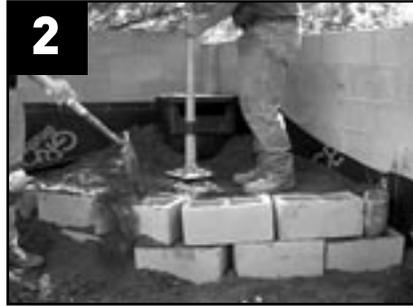
**2** Use soil excavated from the pond to create a runway for the waterfall. A retaining wall of blocks can be used to provide shape and underlying structure.
