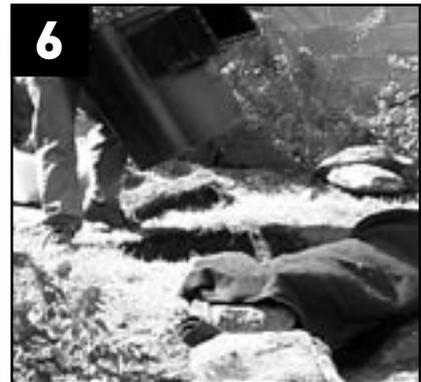
Place the Skimmerfilter.™ in the hole. Check to make sure the intended water level meets the skimmer ¾" inches below the top of the neck. Adjust up or down by adding or removing dirt.
