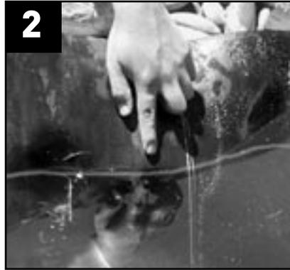
With the pond full, mark position of water level on the liner at the Skimmerfilter.™ location with white chalk.
