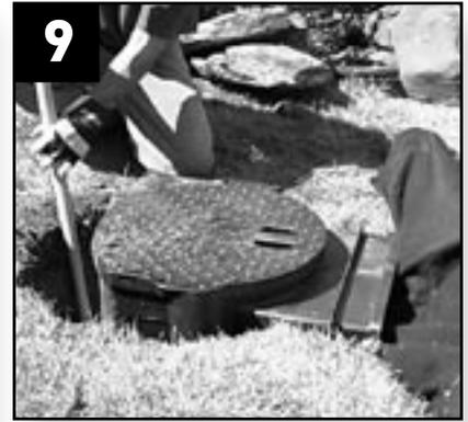
Backfill around the Skimmerfilter™ with the lid in place. Use moist sand or pea gravel or, if unavailable, gravel and loose soil (free from clumps). Hand pack every two or three inches. Do not over compact. Lightly moisten the backfill to aid in settling.
