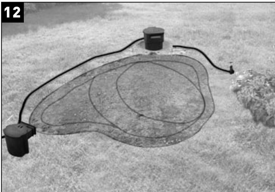
**12** Direct filter drain hose to drainage area. Slope it so water will flow freely during filter cleanings.
