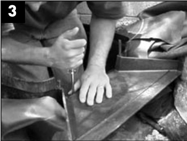
**3** Insert and gently tighten the four large sheet metal screws into the holes in the waterfall weir. Do not over tighten.
