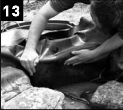
**13** Position pond liner over the Skimmerfilter™ mouth and hold it in place. Smooth liner free of wrinkles and folds. Wipe clean.
