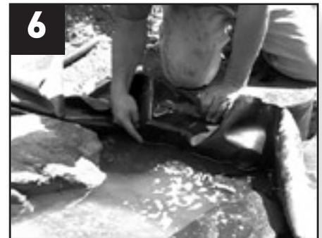
6 Check to make sure the water level meets the skimmer 3/4" inches below the top of the neck. Adjust up or down by adding or removing soil.
