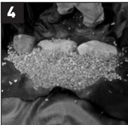
4 Fill behind rockwork with  $\frac{3}{4}$ " - 1 $\frac{1}{2}$ " stones.
