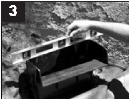
**3** Place the Waterfall Weir™ and level the unit front to back and side to side.
