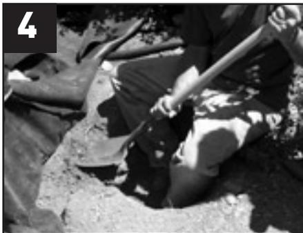
4 Dig a channel 7" below the water line, measuring 15" wide, from the hole to the pond. The Skimmerfilter.™ neck rests on this channel. Compact and level the bottom of excavation. Do not dig too deeply or the soil may settle unevenly.
