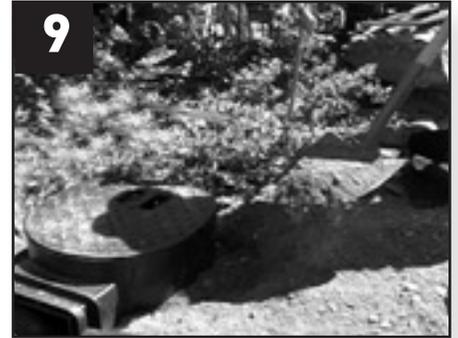
Backfill around the Skimmerfilter™ with the lid in place. Use moist sand or pea gravel, if this is unavailable, use gravel and loose soil (free from clumps).
