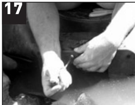
17 Use a #3 Phillips head screwdriver to install screws halfway into all four corners. Install the remaining screws halfway. Tighten top, bottom and sides alternately by hand until screw heads are flush to create a watertight seal.
