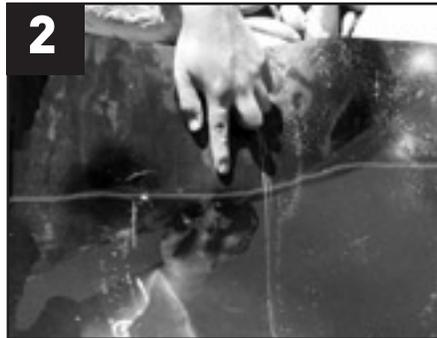
2 With pond full, mark position of water level on the liner at the Skimmerfilter.™ location with white chalk.
