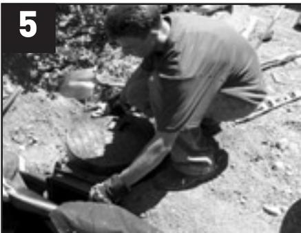
5 Place the Skimmerfilter.™ in the hole. Verify that the face of the Skimmerfilter.™ is flush with the back wall of the lined coping shelf.
