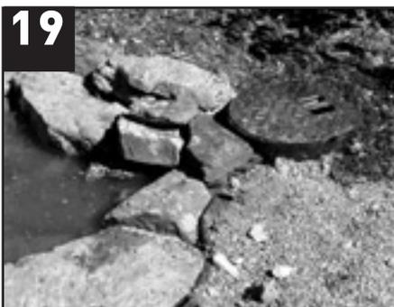
19 Hide the Skimmerfilter™ from view by extending the coping shelf rockwork to both sides of the Skimmerfilter™ opening. Place a flat rock across the Skimmerfilter™ neck.
