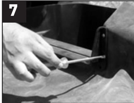
7 Attach liner bracket and liner to waterfall weir by installing 4 tack screws **halfway** into each corner. (Front of seal has recessed screw holes.)
