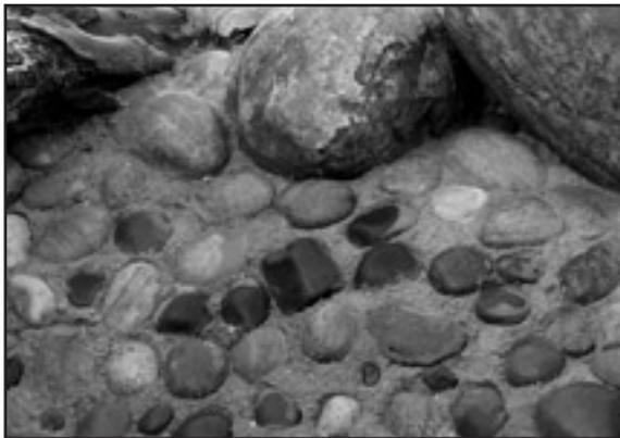
To create a safe, durable, easy-to-clean decorative rock bottom pond, press river stone halfway down into a fresh 2" layer of cement on the shelves. Build up and stabilize vertical stone walls with mortar.
