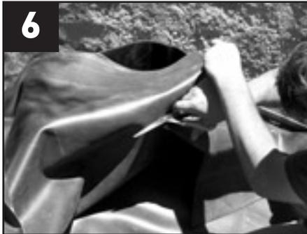
6 Cut away the liner to the shape of the opening.
