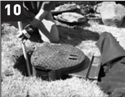
Hand pack every two or three inches. Do not over compact. Lightly moisten the backfill to aid in settling.
