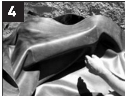
**4** Place liner over the face of the waterfall. Leave a moderate amount of slack in the material.
