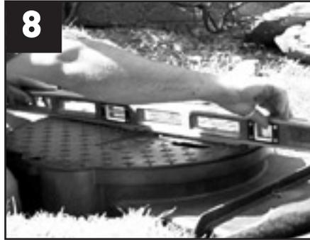
Level the unit front to back and side to side. Dig the front of the hole 1/4" deeper than the back to compensate for settling. **Check water level once again.**
