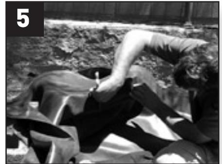
**5** Mark position of the weir opening by rubbing the liner with a hard object such as a screwdriver or a blunt scissor edge.
