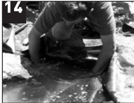
14 Position pond liner over the Skimmerfilter™ mouth and hold it in place. Smooth liner free of wrinkles and folds. Wipe clean.
