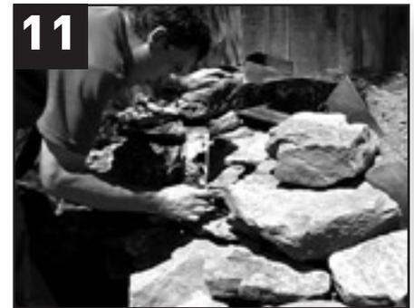
11 Black foam fills voids in the rockwork and forces water to run over the rocks instead of beneath and between them.
