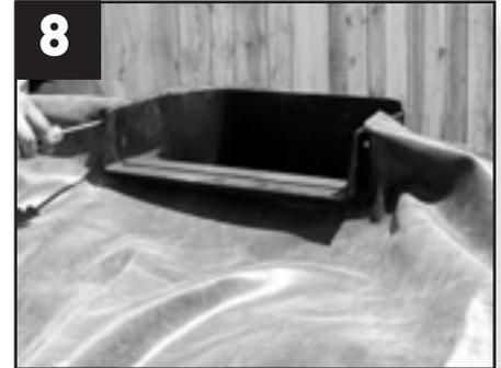
8 Next, install the remaining screws halfway. Tighten all screws evenly **by hand**, until flush with the faceplate.
