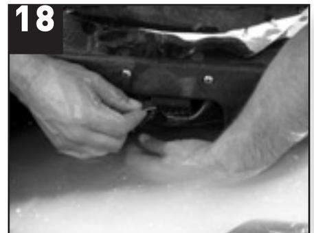
18 After the faceplate is properly tightened use a knife to trim the liner inside the mouth of the Skimmerfilter™.
