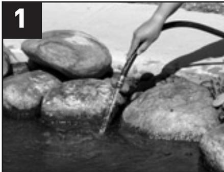
1 Fill the pond with water to accurately determine water level on all sides before installing the Skimmerfilter.™ Water level should hit partway up the coping stones. Verify that the water level is a few inches below the edge of the liner on all sides.
