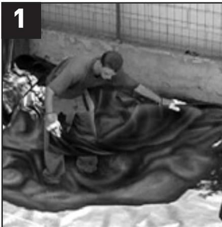
1 Place scrap underlay to protect the liner from abrasion and sharp edges.
