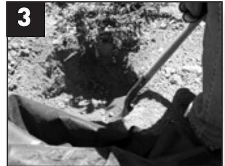
3 Dig a hole for the Skimmerfilter.™ in the previously determined spot. Place the hole 4" back from the coping shelf, measuring 24" across, with a depth of 14" below the marked water line.
