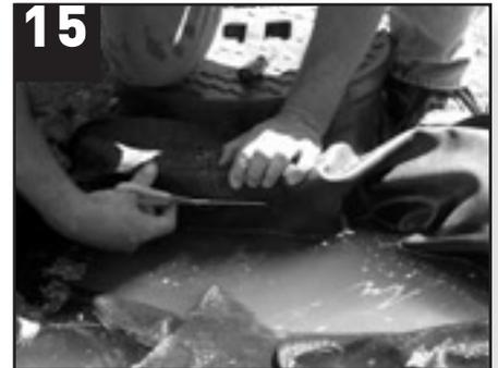
15 Make a 3" wide incision through the centered liner 3/4" below the top of the Skimmerfilter™ opening.
