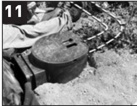
Dig a trench for the kink free hose to the back of the Skimmerfilter. Extend this trench so that it connects to the waterfall weir.
