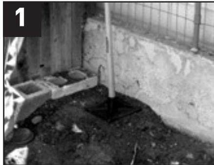
**1** Level the soil in the area where the assembly is to be placed. Use blocks to add height to the waterfall.
