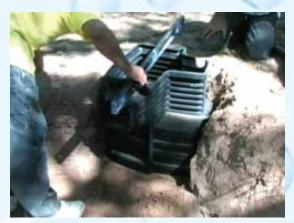
Level the pocket in all directions. Establish the water level for the pond, then the proper placement and height for the skimmer.
