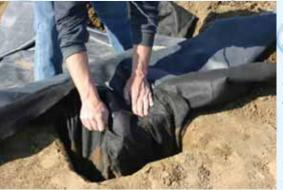
Fold the liner and underlayment back towards the pond, to reveal the void spaces created when digging the skimmer pocket. Backfill around the skimmer with soil in 4" to 6" increments. Compact the soil around the skimmer using the end of the shovel or a 2 x4.
