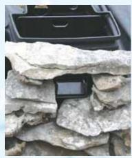
Finish stacking stones up the front of the skimmer. Place the stones on the horizontal ledges to help lock in the skimmer. Use stone to conceal the skimmer door opening.
