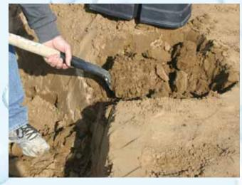
Dig a pocket for the skimmer on the edge of the pond. Over dig the pocket by at least 4" in all directions to ensure plenty of room for the skimmer.
