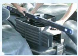
Set the Eco-Series skimmer in the pocket. Double check to make sure it is level in all directions.
