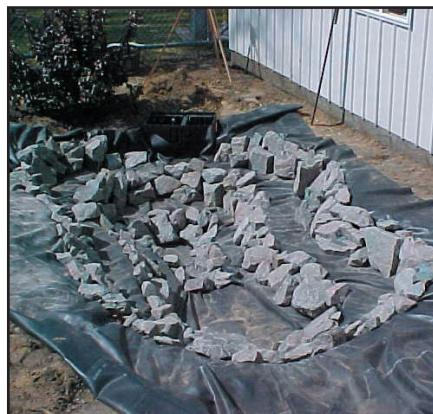
When placing rocks, start in the middle and work outward.
