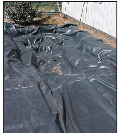
*Installing the liner... Be sure to leave a few extra inches of liner in the pond. These small wrinkles will be covered by the stone and will allow the liner to stretch into place when the pond is filled with water.*
