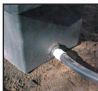
After both bulkheads are installed and the second hole is plugged, apply silicone to the PVC male adapter and turn into the bulkhead fitting. Be sure both pipe and fitting are free of dirt, then apply PVC primer to both followed by PVC glue. Insert pipe into fitting and allow to set for several minutes before burying.
