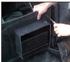
Be sure to use a large bead of silicone around opening. Hold face plate in place and line up holes with an awl.
