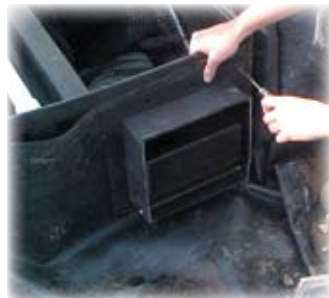
Be sure to use a large bead of silicone around opening. Hold face plate in place and line up holes with an awl. Insert bolts through holes and secure with nut on inside of skimmer.
