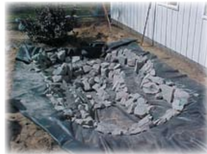
When placing rocks — start in the middle and work outward.
