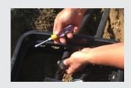
**TLEVEL and Backfill the Junction Valve Box**Check to be sure the Junction Valve Box is level and flush with the ground's surface, then backfill around the Junction Valve Box.
